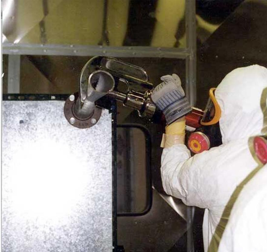
Figure 14. Mega Tech Blade Plunging Cutter being used to cut 2.5 inch (6.35 cm) OD pipe.
