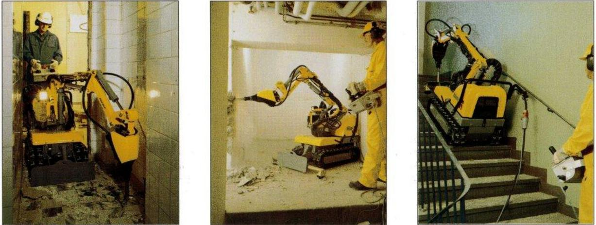
Figure 21. Brokk Demolition Machine (Model 40) equipped for remote control impact demolition.
