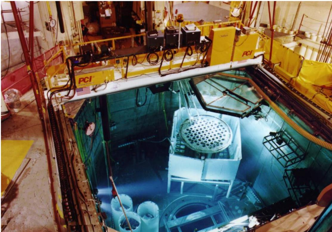
*Figure 1. Yankee Rowe flooded Reactor Cavity with Manipulator Bridge running on rails on both sides of the pool and Reactor Internals Segmentation Cubicle sitting on the bottom of the pool (with Upper Internals inside it).*
