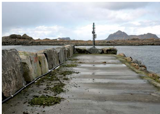
Figure 7-15 Example of concrete foundation and cable attached to breastwork. (Bodø and Steinesjøen. Photo: Norwegian Coastal Administration).
