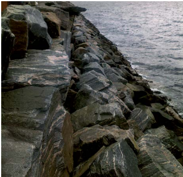
Figure 8-14 Example of well-executed interlocking surface in protected areas: the blocks are sitting with a good angle and are interlocked well with each other. This is an acceptable method for protected areas, where the waves are moderate. For more exposed areas, a bit more rough surface with greater unevenness would be preferable. The crown wall at the top consists of free-lying blocks that are not secured, something that is acceptable here. (Vikan, Kristiansund. Photo: Norconsult).
