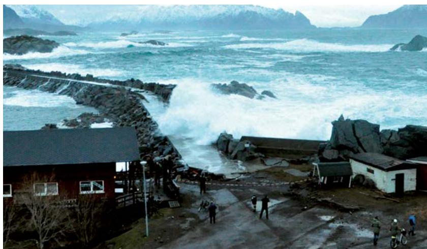
Figure 7-14 Picture from Kabelvåg during the storm Berit, which shows that the police have blocked off the breakwater. (Photo: Bjørnar Larsen, Lofotposten).
