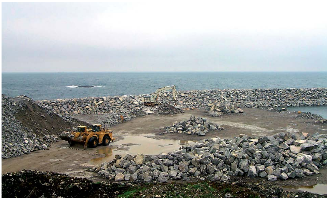
Figure 8-1 Intermediate storage of rock requires large areas, but is a good investment because it makes it easier to attain the desired quality for the finished product. (Sirevåg. Photo: Sintef).
