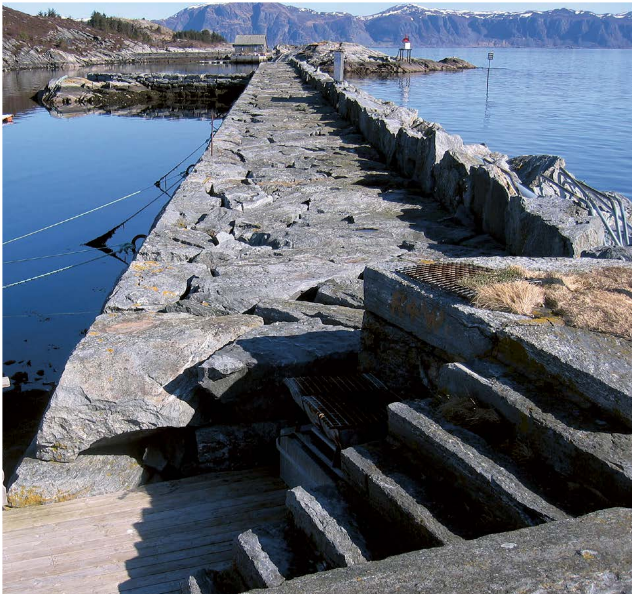
Figure 12-1 Part of the breakwater at Silda, Municipality of Vågsøy. The older part was completed in 1889. The structure is a good example of how regard was paid to a certain degree to the architectural style and use of material when further expanding the breakwater.
