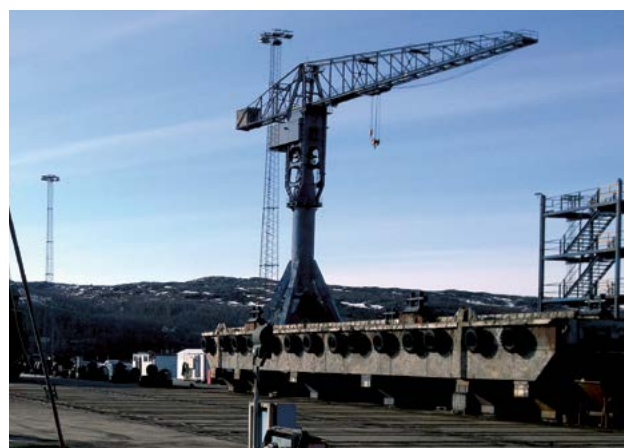
Figure 3-14 Example of floating wharf of unknown origin (Kirkenes, Norconsult). The structure is large and heavy enough that it will attenuate waves of up to approximately 4-5 s periods.
