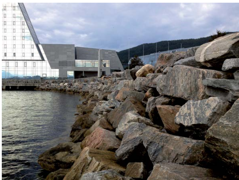
Figure 8-7 Example of blocks that are well-suited for interlocking surfaces (and possibly walling) – the blocks have an angular shape and at least one flat side, which enables them to work together well with other blocks. (Molde. Photo: Norconsult).
