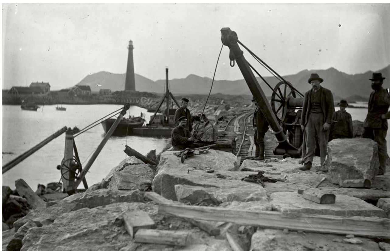
Figure 2-1 Breakwater construction at Andenes in 1902.
