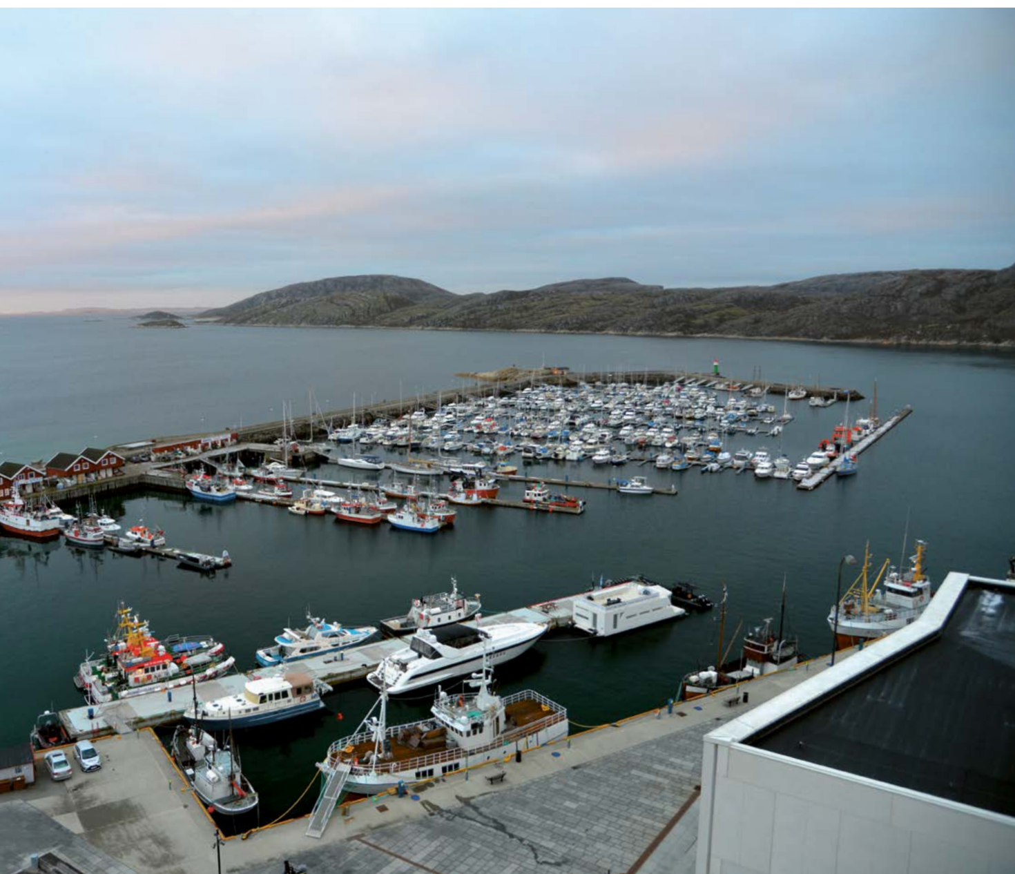
Figure 6-15 A breakwater may have multiple secondary functions. The picture shows the breakwater in Bodø, which, in addition to shielding the harbour basin further in, is an attractive destination for outings and shields the small craft harbour. (Photo: The Norwegian Public Roads Administration).
