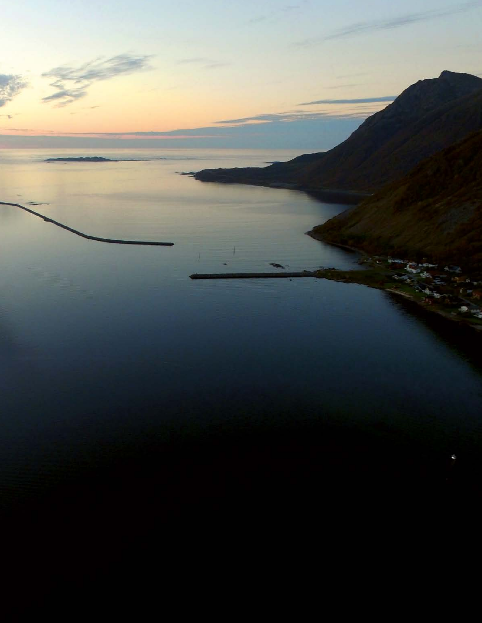
Breakwaters outside Myre Harbour. Photo: Per Aarsleff AS
