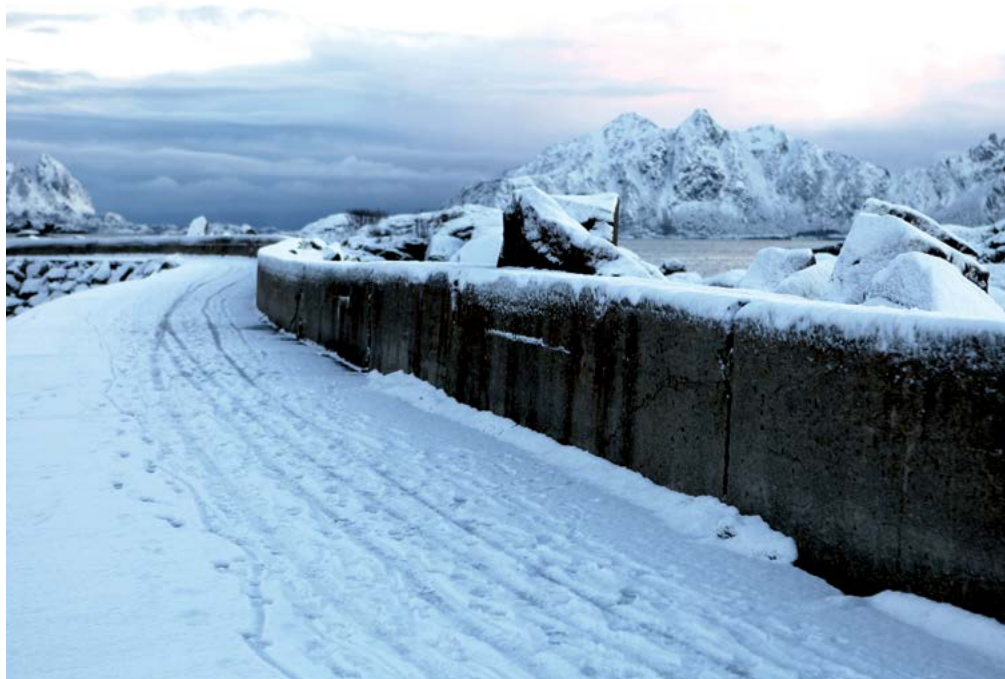
Figure 7-11 Solid crown wall implementation. Upright blocks with back edge reinforcement of concrete. (Svolvær. Photo: Norwegian Coastal Administration).
