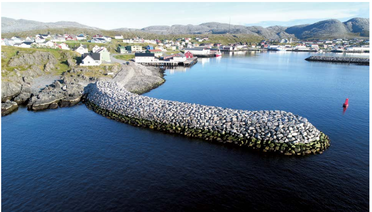
Figure 6-13 Mehamn, Finnmark – round armoured breakwater. (Photo: GeoNord AS).
