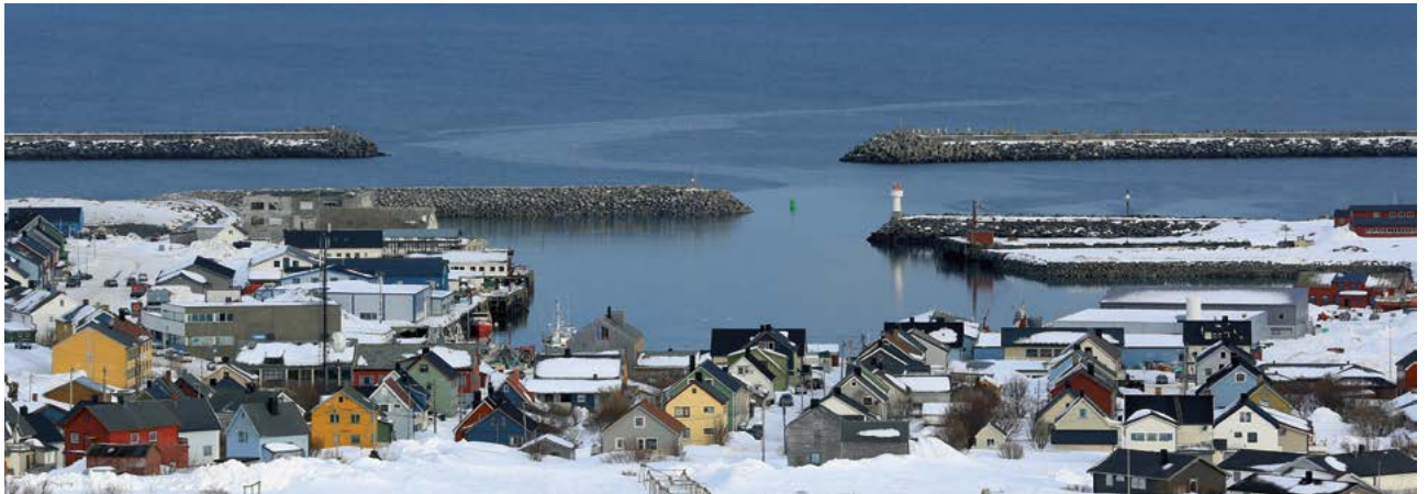
Figure 6-12 Berlevåg, Finnmark. The breakwater is fundamental for the business activity and thus the existence of the fishing village. (Photo: Tore Larsen, Berlevåg).
