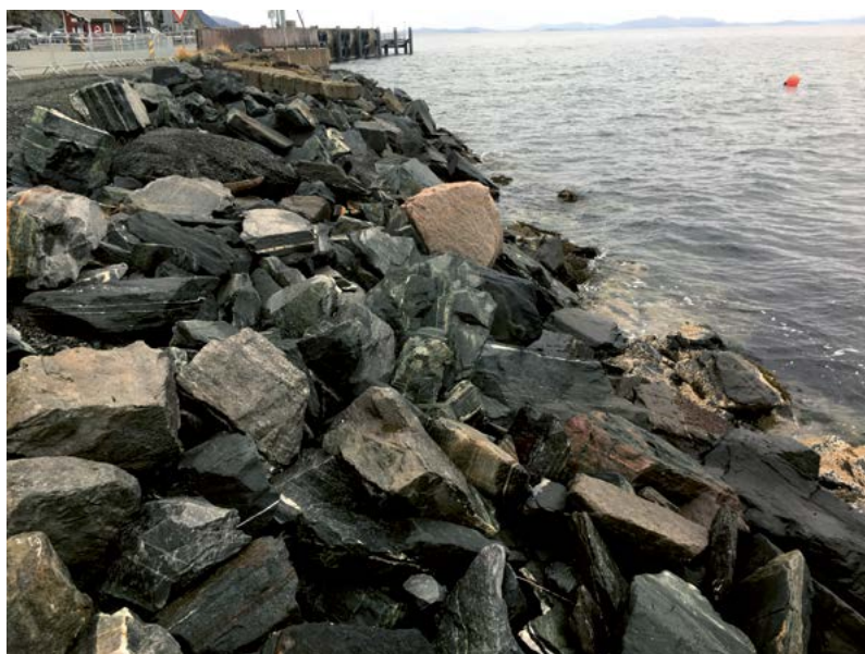
Figure 8-13 Example of construction method "Rubble embankment" from table 3-1. (Photo: Norconsult) MUST NOT BE USED IN BREAKWATER CONSTRUCTION.
