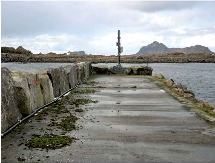
Figure 8-21 Example from Steinesjøen, Vesterålen, where a solid crown wall was built of upright armour units. (Photo: Norwegian Coastal Administration).
