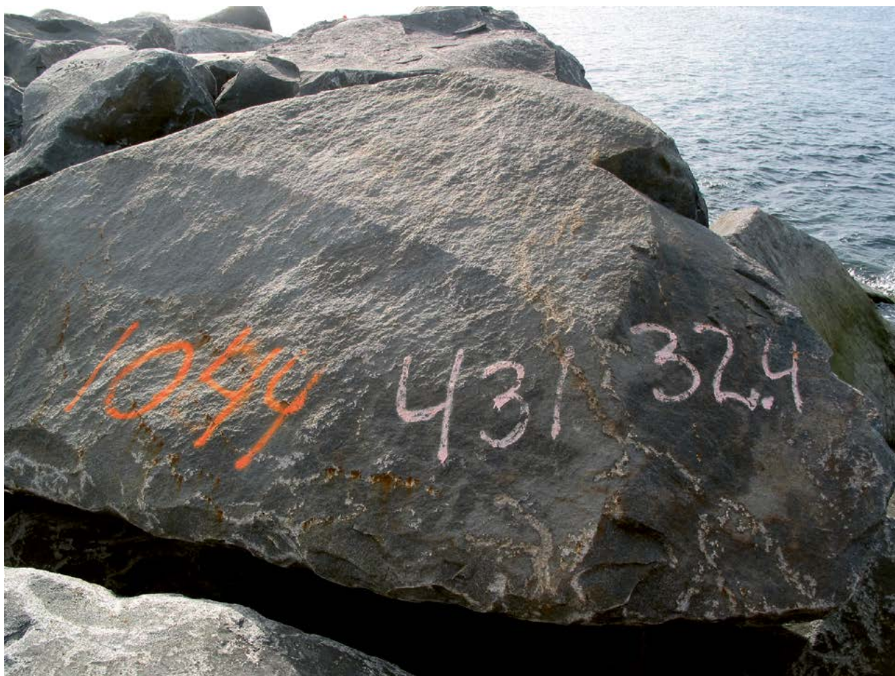
Figure 8-10 For larger structures with strong wave loads, it is relevant to weigh and number every single block and store its position electronically (weight 32.4 tons). (Laukvik. Photo: Norconsult).
