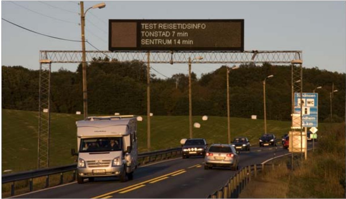
Figure 2: VMS with travel time information at Okstadbakken.
