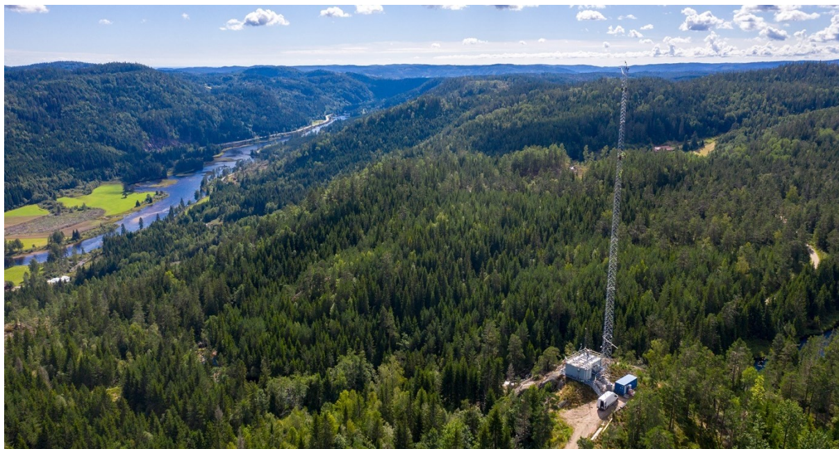
Figure B 2: The Birkenes Observatory is located on top of a small hill with a prominent 75m mast. Photo credit: Kjetil Samuelsen, Fædrelandsvennen.
