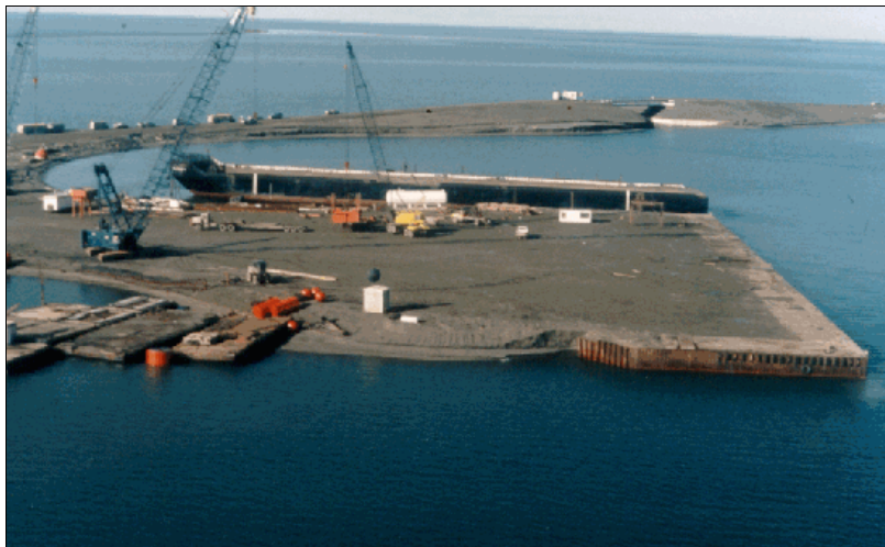
Figure 8 - 11 Man-made solid structure: dock of pilings and sheet metal, Prudhoe Bay, Alaska
