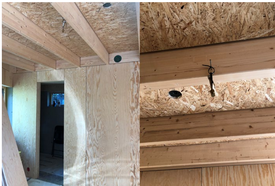
Figure 15. The sampling site with highest concentrations of \alpha - and \beta -pinene. The untreated natural wood materials act as a source for pinene emission to this indoor environment.
