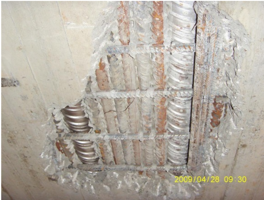
Figur 28 For tett armering (foto: Linda Brateng)
