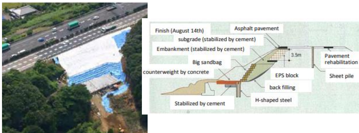
Figur 73. EDO-EPS Method Applied for Rehabilitation of Expressway Hit by Earthquake Central Nippon Expressway. Foto og illustrasjon: EDO
