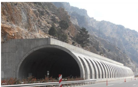
Figur 77. Geofoam blocks applied for energy absorption on rock fall protection tunnel in Turkey (Foto: Courtesy of EPSDER, Turkey)
