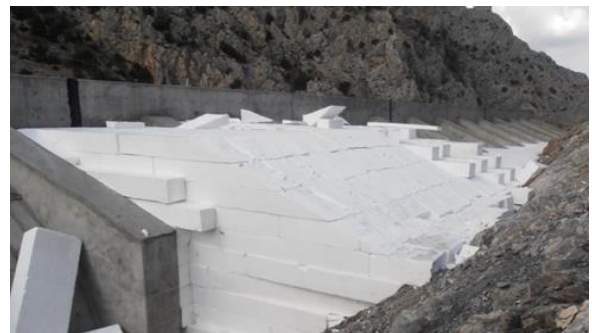
Figur 77. Geofoam blocks applied for energy absorption on rock fall protection tunnel in Turkey (Foto: Courtesy of EPSDER, Turkey)
