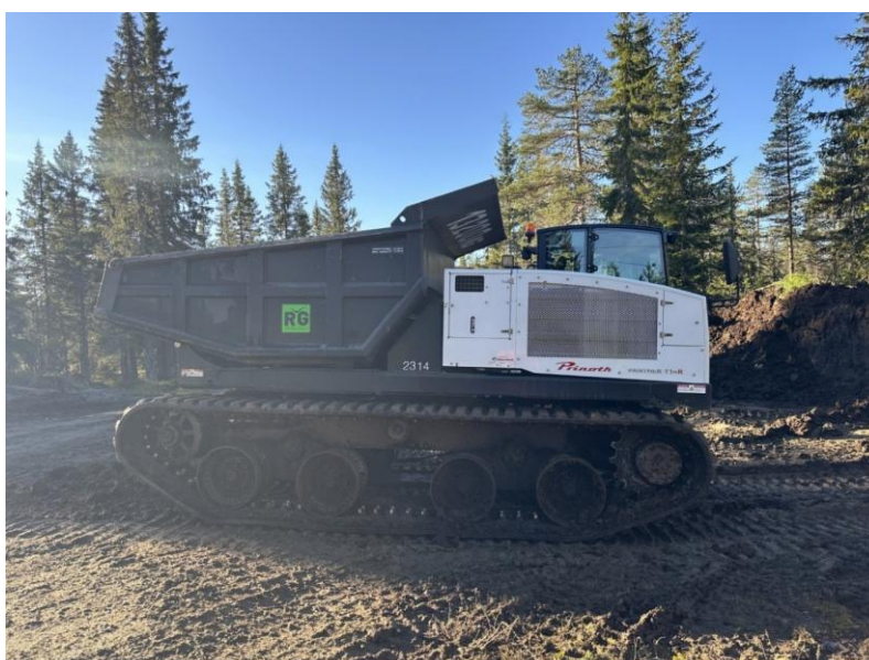
Figur 11: Beltedumper (17 tonn). Foto: Even Stensrud
