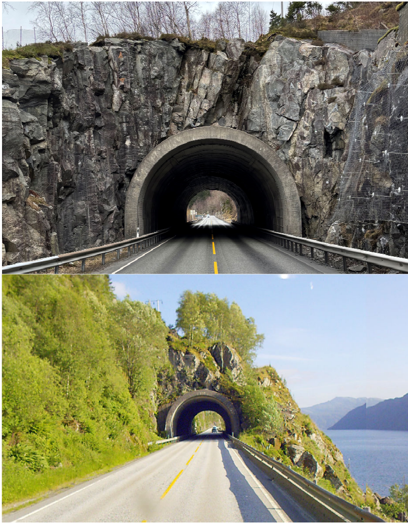
Fig. 16 The Kleinslåt Tunnel on highway E16 in Vaksdal municipality between Bergen and Voss. The tunnel has a length of 55 m and was opened in 1970. A typical example of a road tunnel excavated according to principles adopted from hydropower development. Rock supported with rock bolts and some shotcrete. Top: Viewed from the south. Bottom: Viewed from the north
