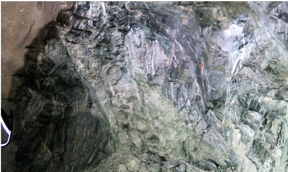
Fig. 9 Chainage 13616 in tube T52 at the E39 Svegatjørn–Rådal project.
