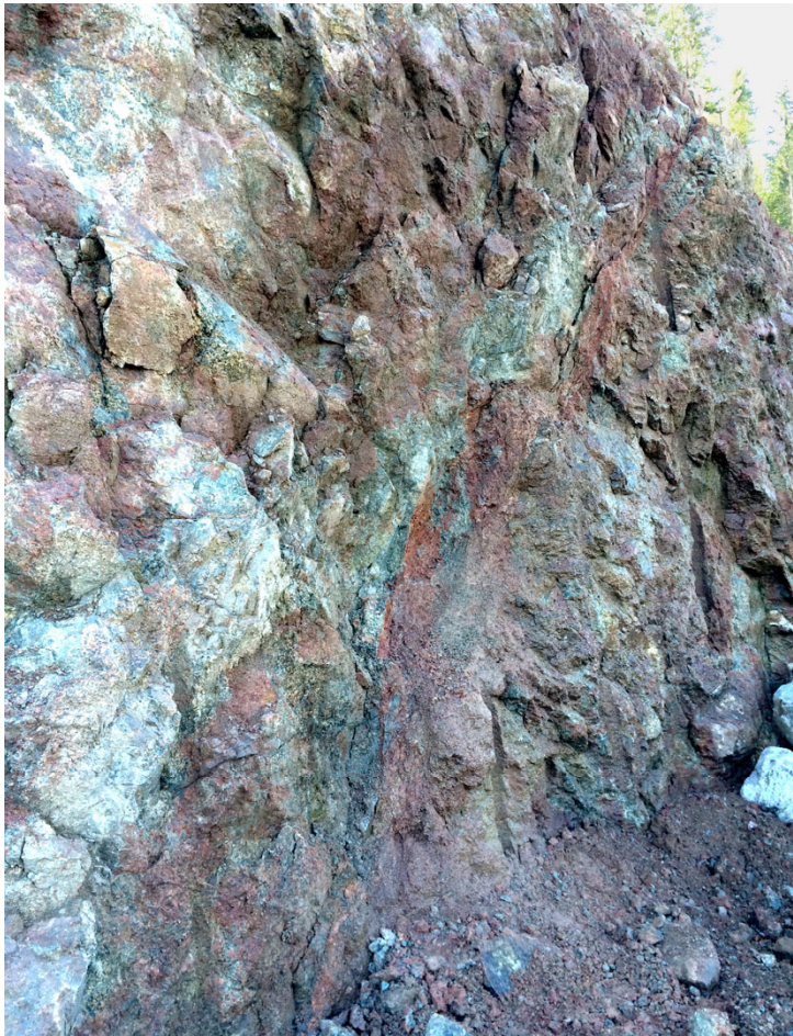
Fig. 10 Road cut just outside the Martineås tunnel at the E18 Bommestad–Sky project close to Larvik
