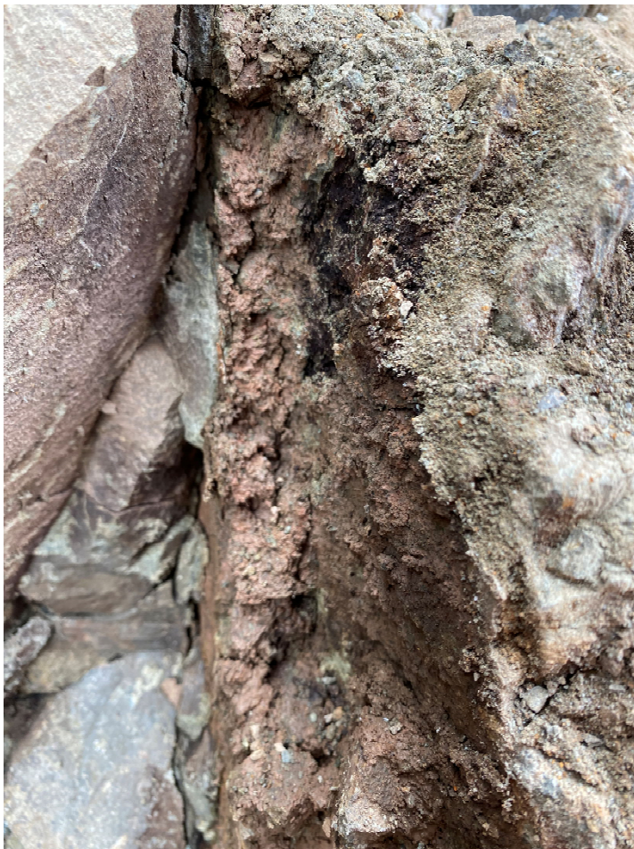
Fig. 7 Detail of the weakness zone shown in Fig. 6.
