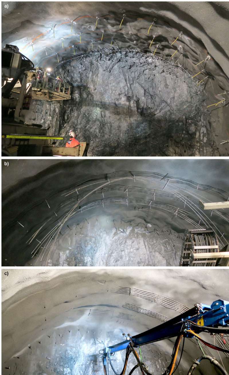
Fig. 19 a) Spiling bolts to support the next blasting round are pre-mounted with steel straps and radial rock bolts. Radial rock bolts for three ribs of sprayed concrete are mounted with thread protectors (yellow). b) A layer of sprayed concrete is applied to smoothen the surface. The spiling bolt mounting is also covered with sprayed concrete to secure it. Pre-bent rebars are mounted in brackets fixed to the rock bolts. c) The ribs of sprayed concrete is sprayed with concrete to form the ribs (Høien 2018)
