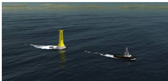
Figure 20. Self-installing gravity base structure (GBS) during towing to site. Source: Seatower, 2011
