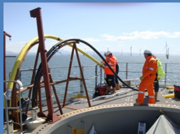
1 cable laying vessel for replacing power cables 11
