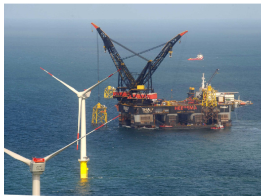
Figure 23. Installation of jacket at the Alpha ventus site with the Thiaf installation vessel. Source: NorWind, 2009
