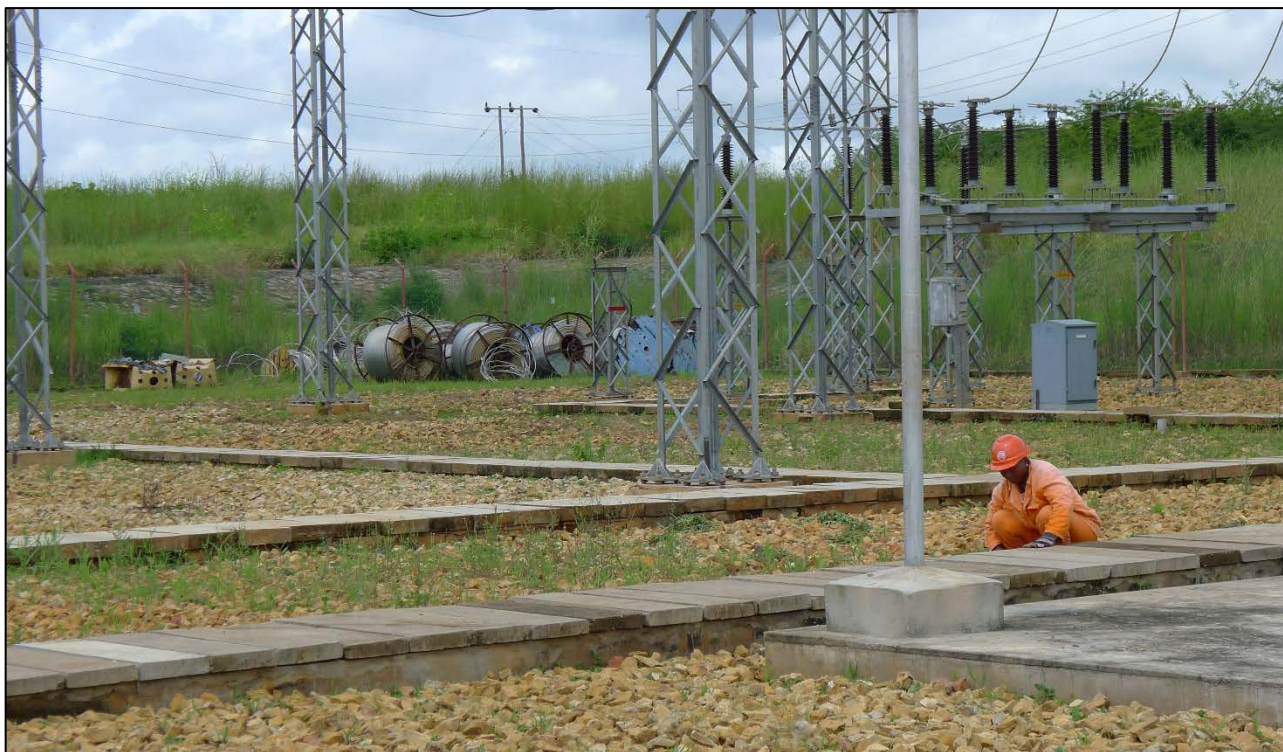
Picture 3. Vegetation clearing at Metoro substation.
