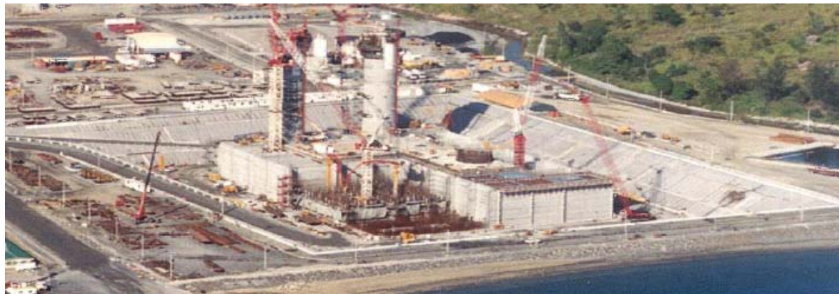
Figur 10. “Purpose built” tørrdokk
