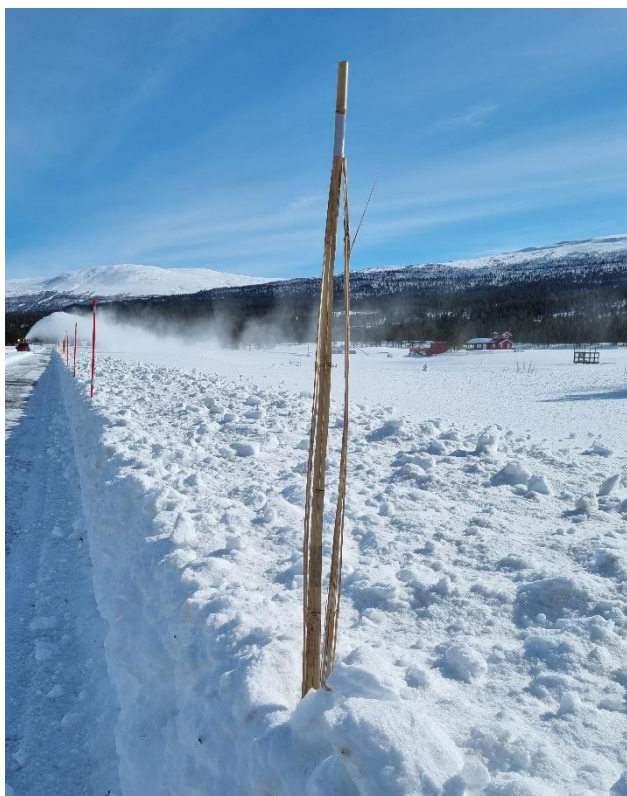
Figur 42: Spjæret Bambus 26/28 mm.
