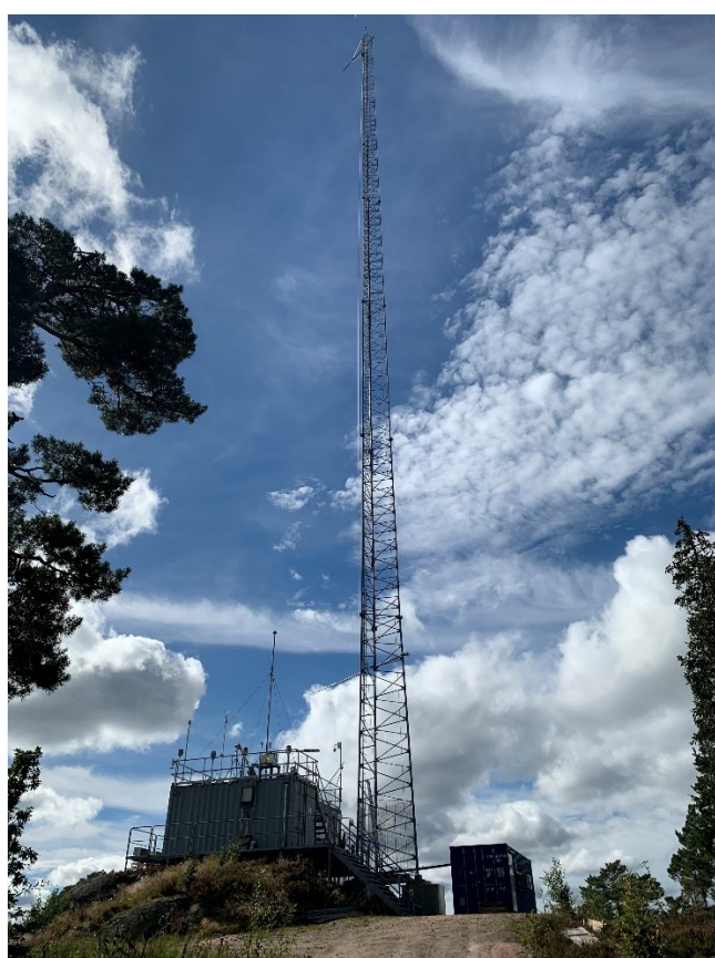
Figure 3: The two atmospheric observatories included in this programme, Zeppelin above and Birkenes to the left. A 75 m tall mast was installed at Birkenes in 2020.
