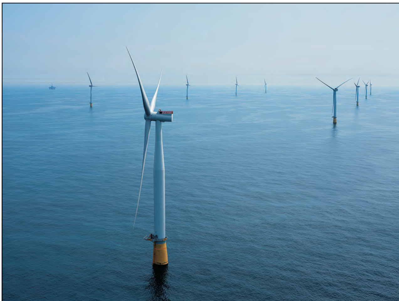
Figure 5.8 Floating wind turbines in the Hywind Tampen wind farm.
