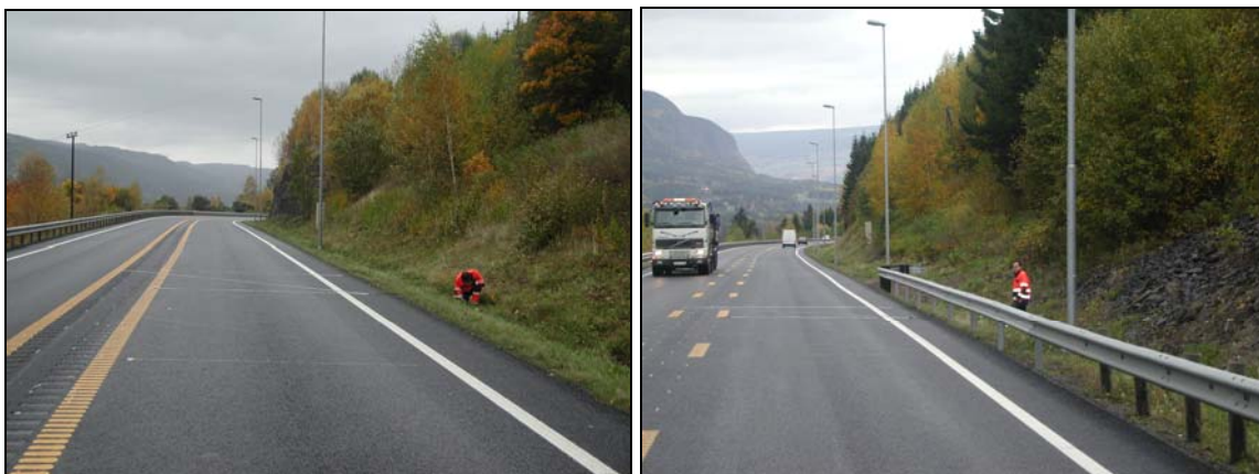
Visual central reserve with different road markings
