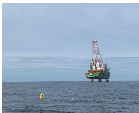
Figure 50: SmartPAM real-time bioacoustics buoy in operation during the construction of Saint-Nazaire offshore wind farm. Source: Quiet-Oceans
