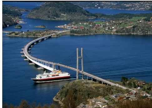
Area 2. Floating bridge Nordhordlandsbrua 60°31'21.4"N 5°16'10.8"E
