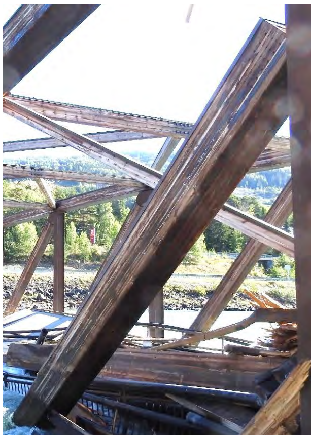
Figur 139 Knutepunkt OG16A, feste for diagonal 7A
