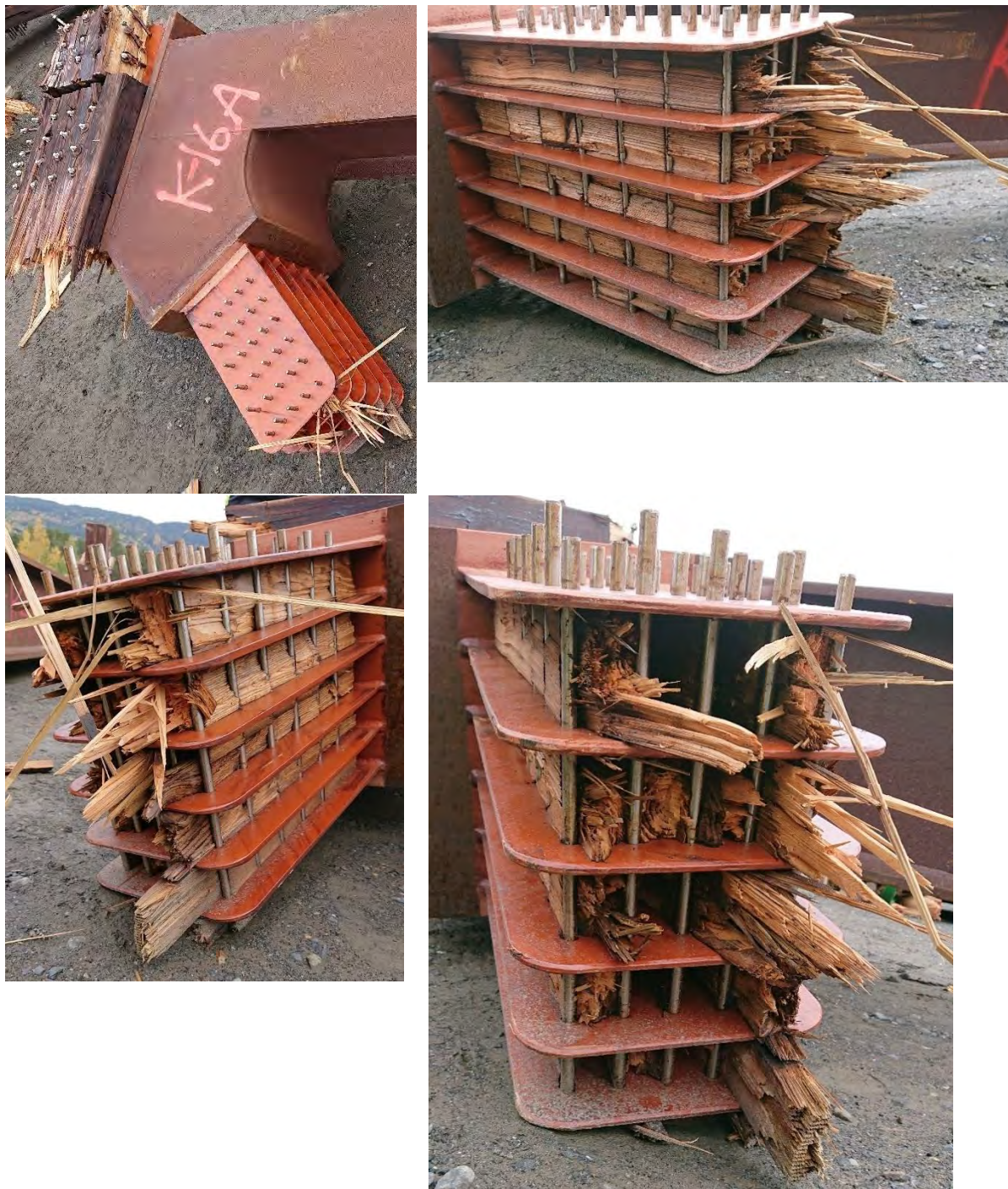
Figur 140 Knutepunkt OG16A, feste for diagonal 7A
