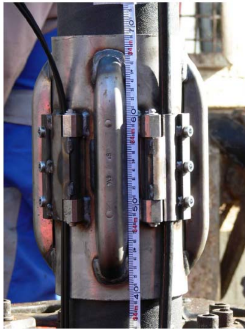
Figure 4.2: Permanent installation of cable behind casing. DTS cable on left hand side. Henniges et al. (2008), GFZ Potsdam
