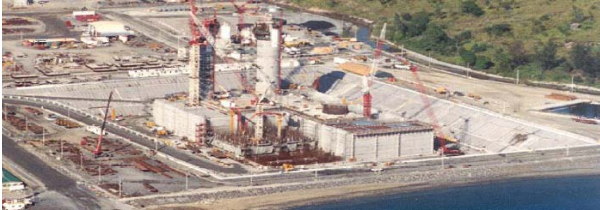
Figure 11 “Purpose built” dry dock [13].
