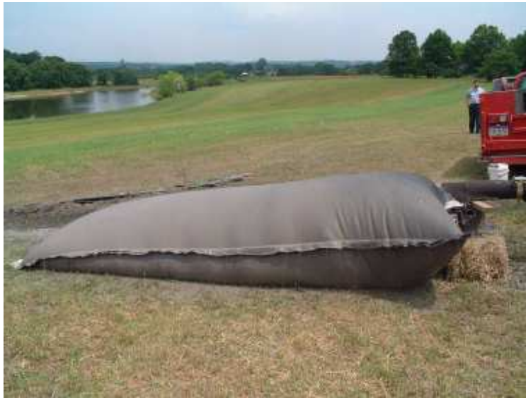
Figur 22. Geotekstilpose for muddermasser
