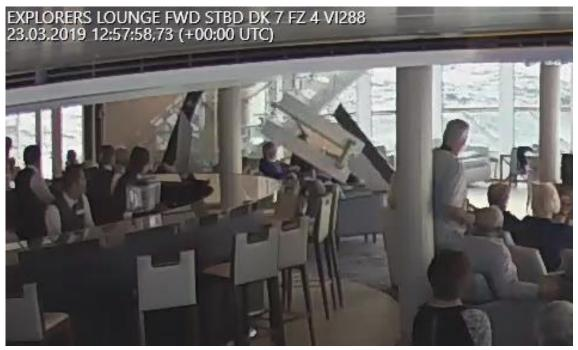
Figure 10: Ceiling plates falling down in the Explorer's Lounge at the time of the blackout. Photo: CCTV
