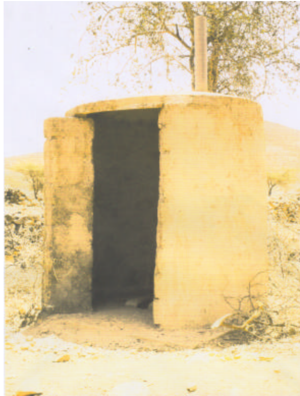
Construction of Model latrines in Shebah and Demas have contributed greatly to reduce sanitation and health problems. The latrine in the picture is a model specified by the MoH.
