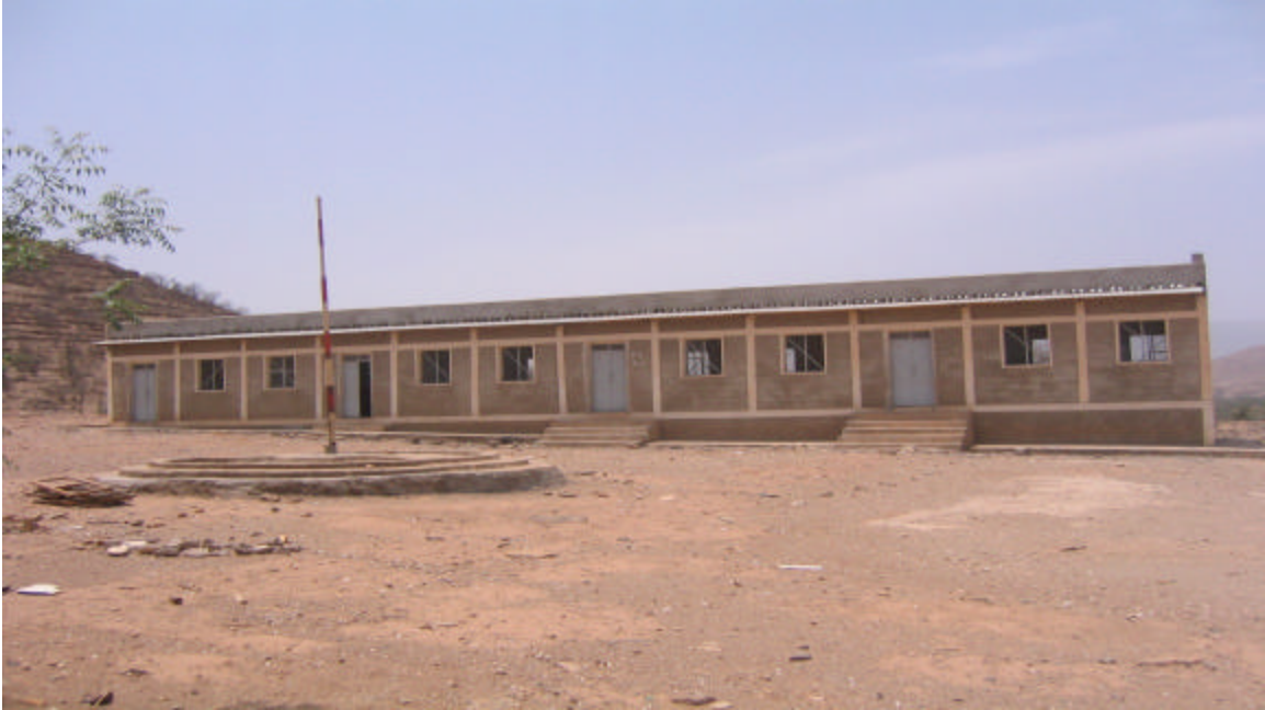
Full renovation of Demas primary school after it was damaged by sand storm.
