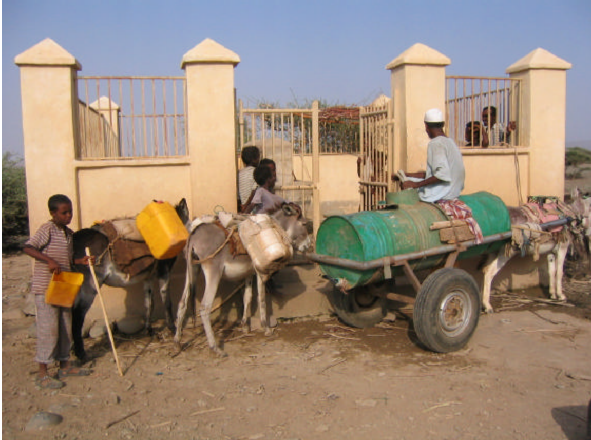
Fenced and protected water facility in Shebah: long distance and unclean water are history. A donkey pulled cart waiting to carry many liters of water in one go!!! Could this be a relief to commuting several times to fetch a few liters of water?
