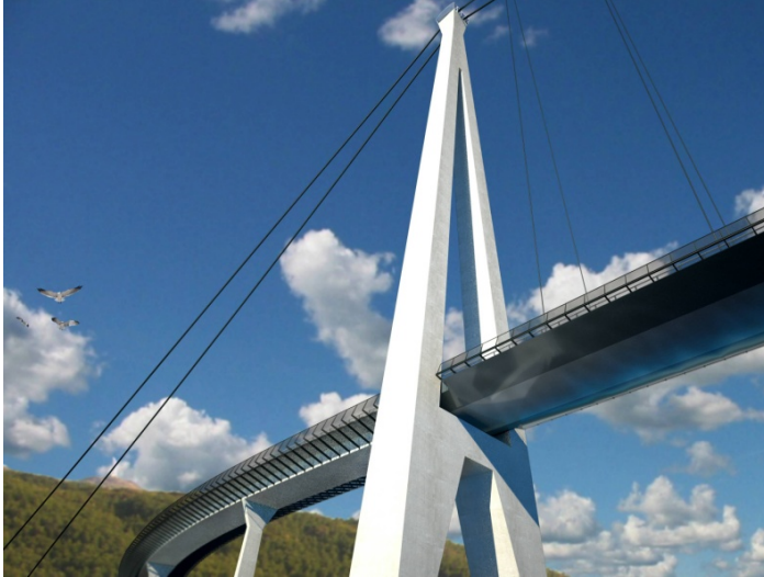
Figure 11: Illustration of Hålogalandsbrua (cowi/Satatens vegvesen)
