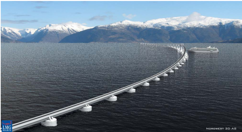
Figure 12: Concept of Floating bridge crossing Björnafjorden(Lmg Marin)
