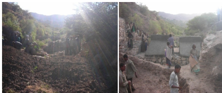
Photo: Water harvesting check dam during construction
