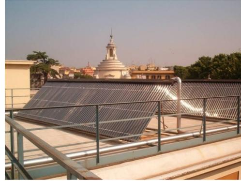
**Figure 2. Installation with vacuum tube collectors. Foto: Thermomax/ ESTIF**
