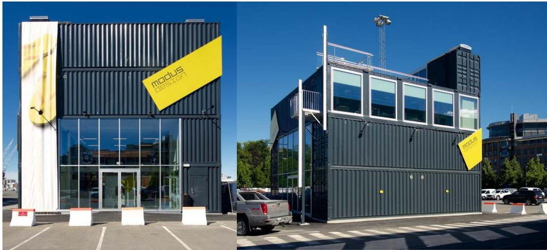
Figure 4.2: Containerised structure like the one planned for Oslo City Hub. Offices belonging to Modus Design AS at Filipstad in Oslo. Photo: Nils Petter Dale. Reprinted from: mmw.no
