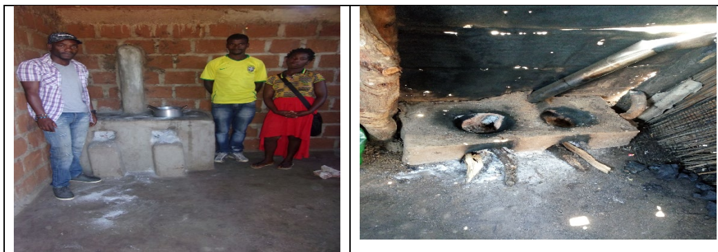
Fig. 4 – Fixed improved Cook Stove: On the left good example and on the right, rain water comes in and destroy the cook stove
