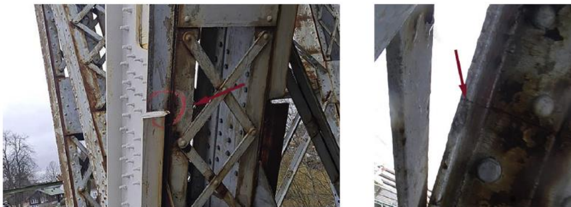
Figure 13: Detected damage [8]. The damage is a fatigue crack that has occurred at the bottom flange (and part of the web) of the angle profile shown in the picture.
