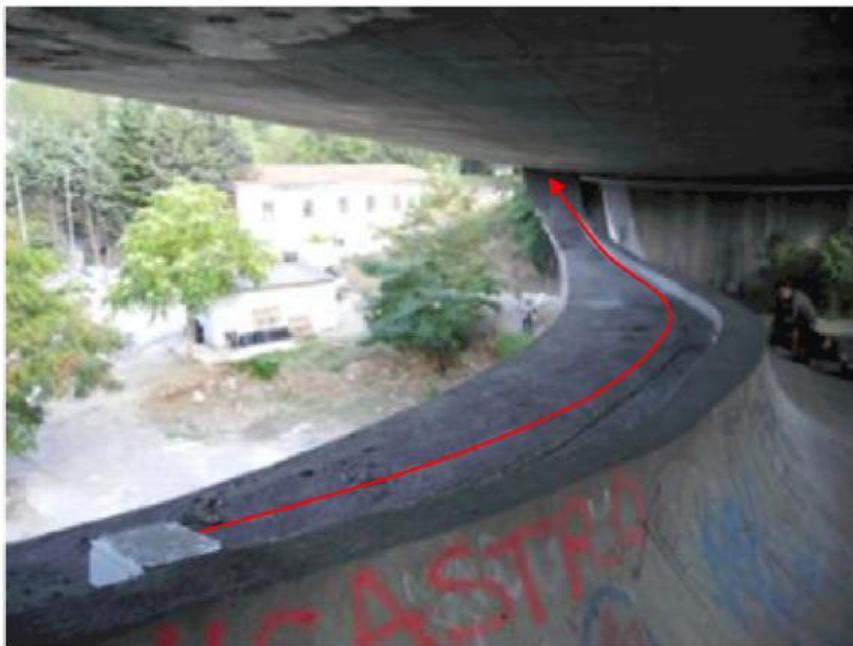
Figure 19: Instrumentation of optic fibers [14].
