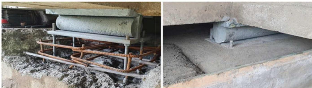
Figure 10. Damaged support (left) and repaired support (right). [7]. (courtesy of Kjetil Sandvik Sletten/Statens vegvesen)
