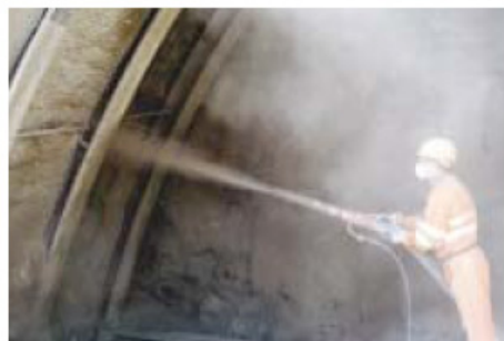
Fig. 2.1: Dry shotcrete application
