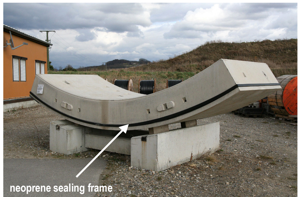
Fig 3.7: Prefabricated concrete segment (tubbings) with a neoprene sealing frame
