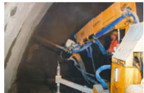
Fig. 2.2: Wet shotcrete with robot
