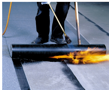
Fig 3.3: Application of a Polymer-bitumen membrane
