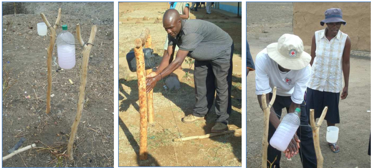
Photos 1, 2, 3: The 'Tip-Tap': a very simple but effective hand-washing structure (l) made from locally available materials and suitable for use at institutional level (c) or in homesteads (r).
