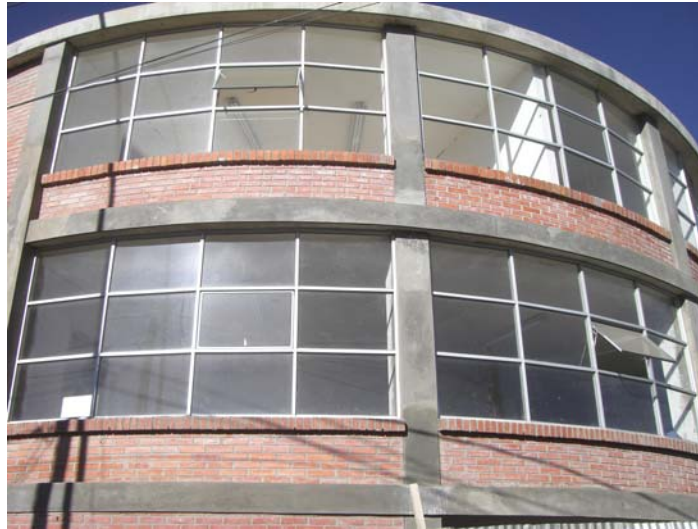
Figure N° 2 Construction of the CRVIR headquarters in El Alto, June 2009
