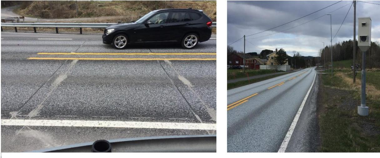
*Figure 1 ATK Piezo cables and camera unit*
