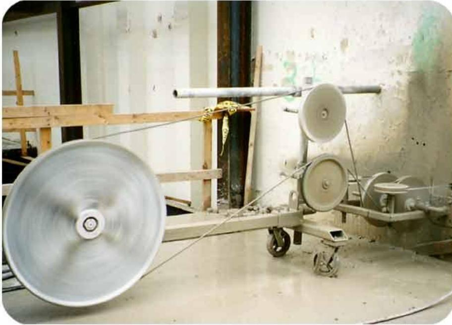
Figure 19. Typical Wire Saw drive in action cutting a section of wall.
