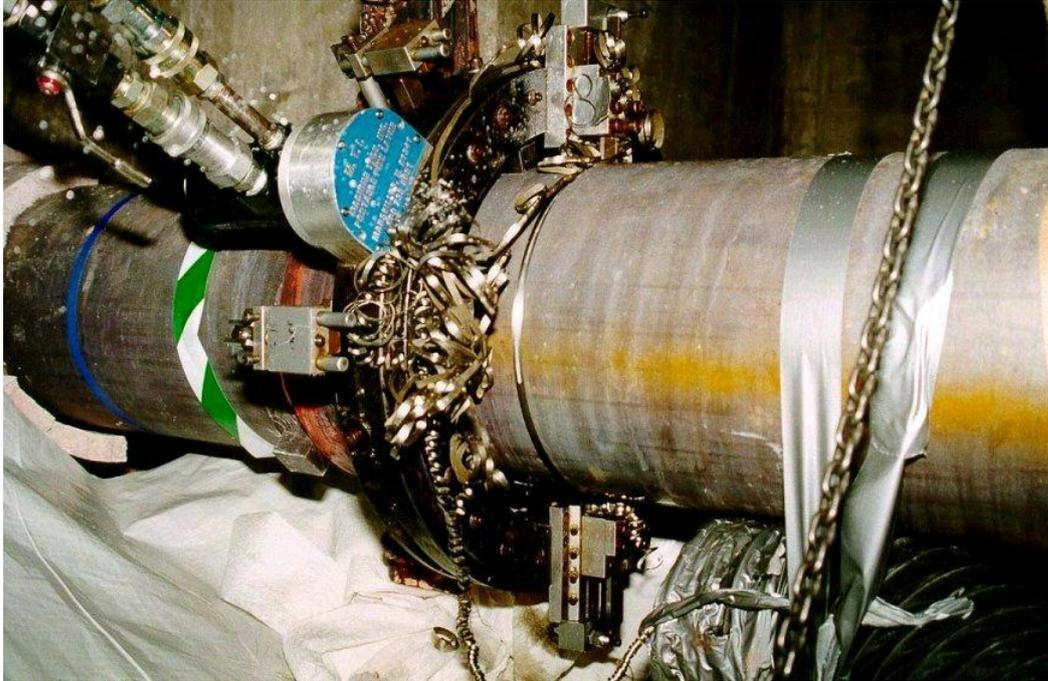
Figure 10. "Clam Shell" Pipe Cutter in Operation.
