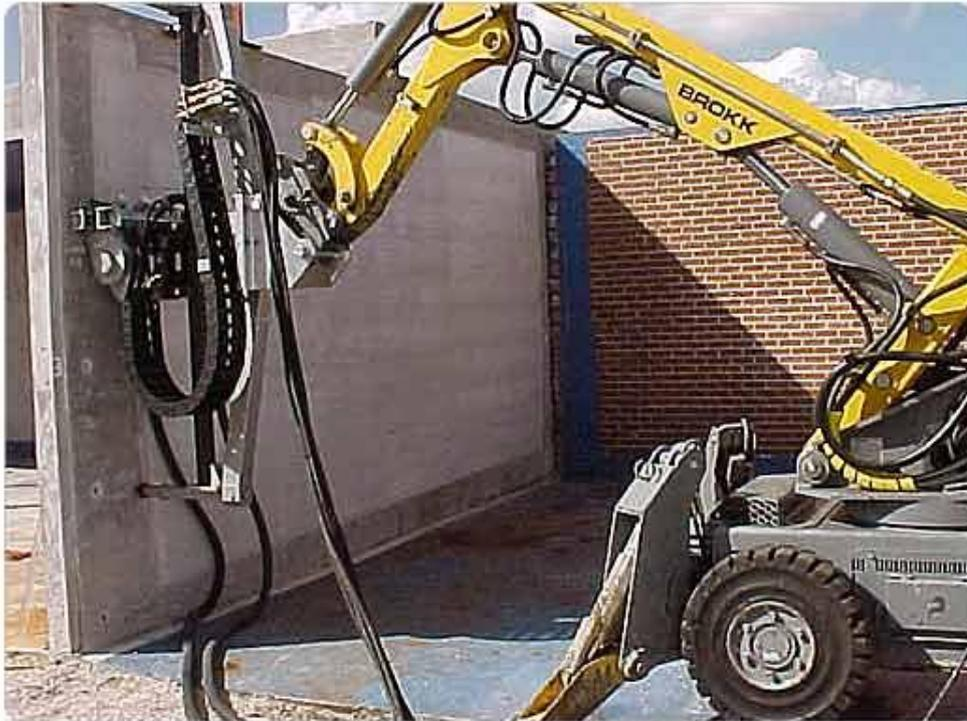
*Figure 18. Floor Shaver mounted on Brokk 250 for wall decontamination.*
