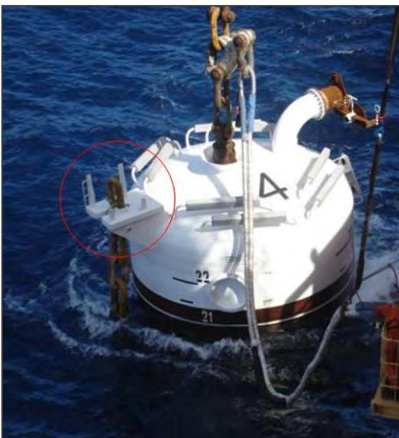
Figure 9-9 Installation of anchor with bottom chain connected at anchor hang-off table (Photo by Vicinay)
