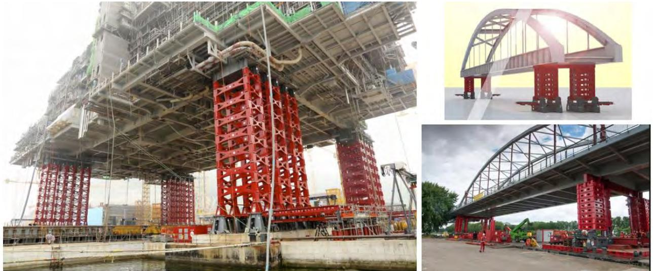
Figure 7-7: Examples of jacking towers (from ALE)
