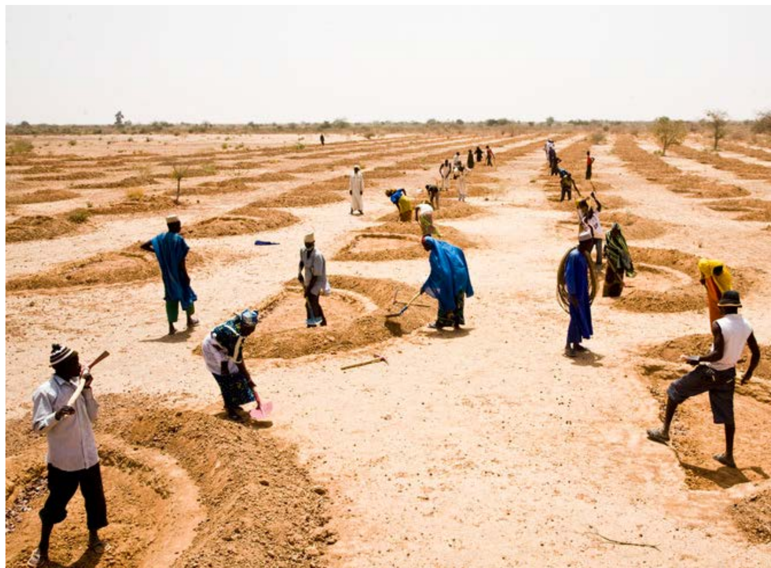
In a region frequently hit by drought, these half-moon structures can play a significant role in preventing future disasters. They are designed to preserve the rain water when it next rains, refilling the water table and encouraging the regrowth of vegetation. Dosso, 2012. Photo: Fatoumata Diabate/Oxfam/Flickr
