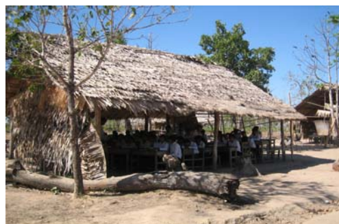
Picture of mini-school built by the community (Source: SCN Basic Education Office, 2008)
