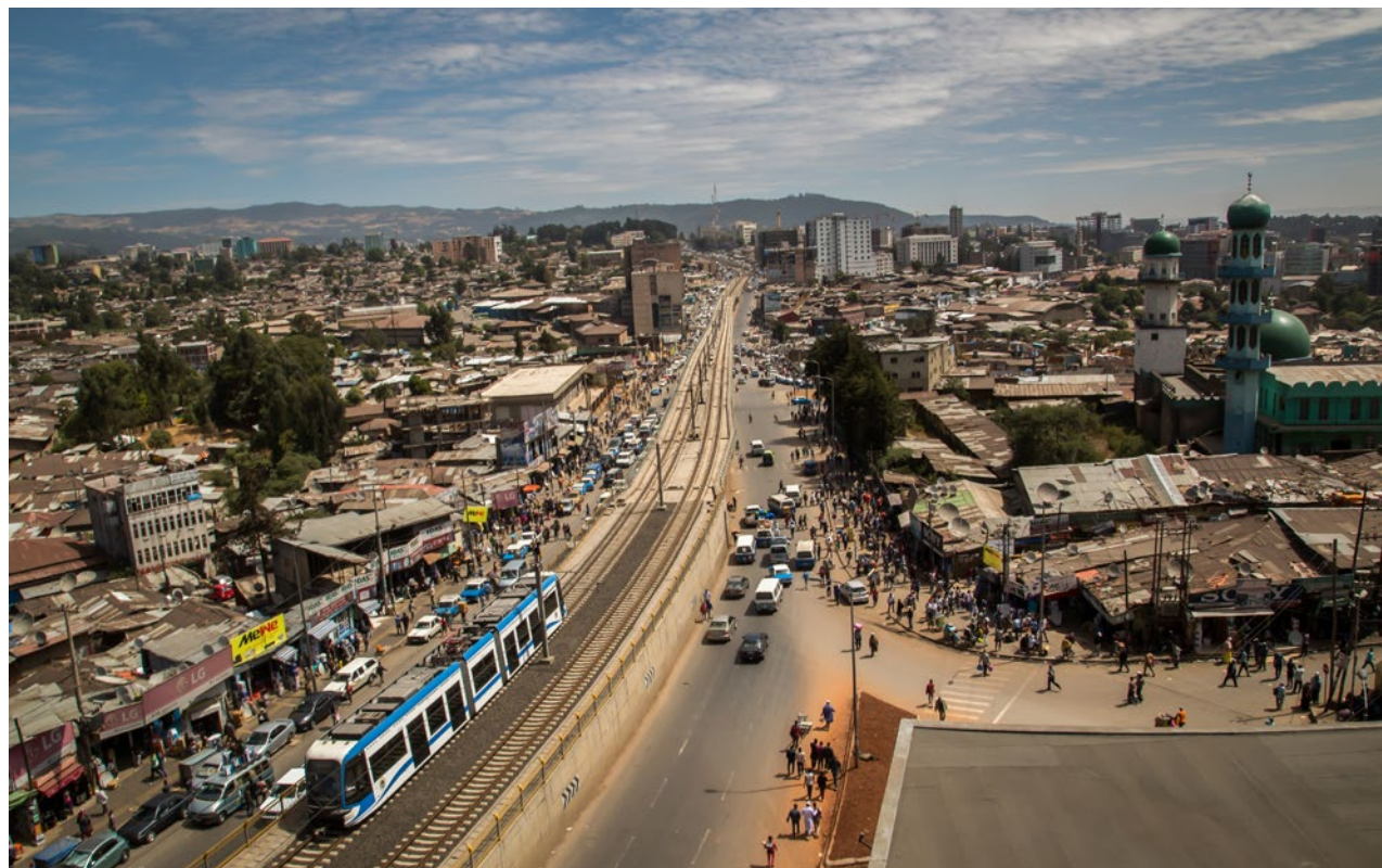
The first line of Addis Ababa's new metro opened in 2015, the first of its kind in Sub-Saharan Africa. Largely funded, constructed and run by Chinese institutions, the train can transport 60,000 passengers per hour, helping to cut the city's greenhouse gas emissions. PHOTO: MULLUGETA AYENE/AP
