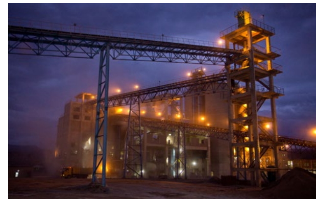
The cement factory in Dire Dawa produces 3,000 tons of cement a day to help meet the demand of the country's building boom. PHOTO: SIMON DAVIS/DEPARTMENT FOR INTERNATIONAL DEVELOPMENT
