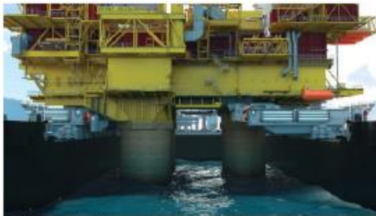
5. All support yokes positioned, upward pressure is accumulated through de-ballasting
