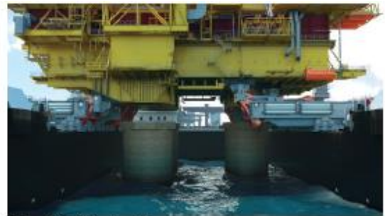
6. Fast lift of the topsides
