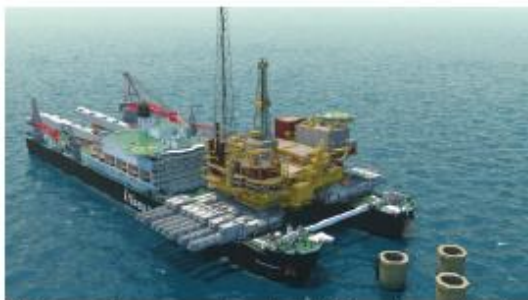
7. The vessel moves away from the platform; the sea-fastening is locked
