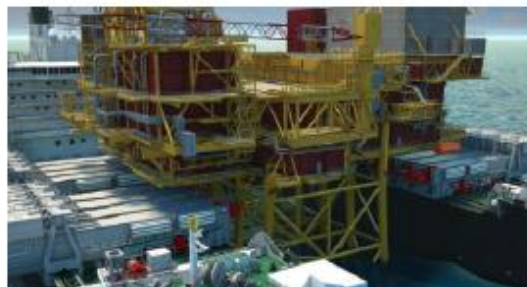
2. The vessel positions itself accurately to connect the horse shoes
