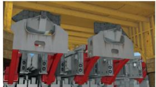
4. The support yokes are positioned at predetermined strong points on the underside of the topsides
