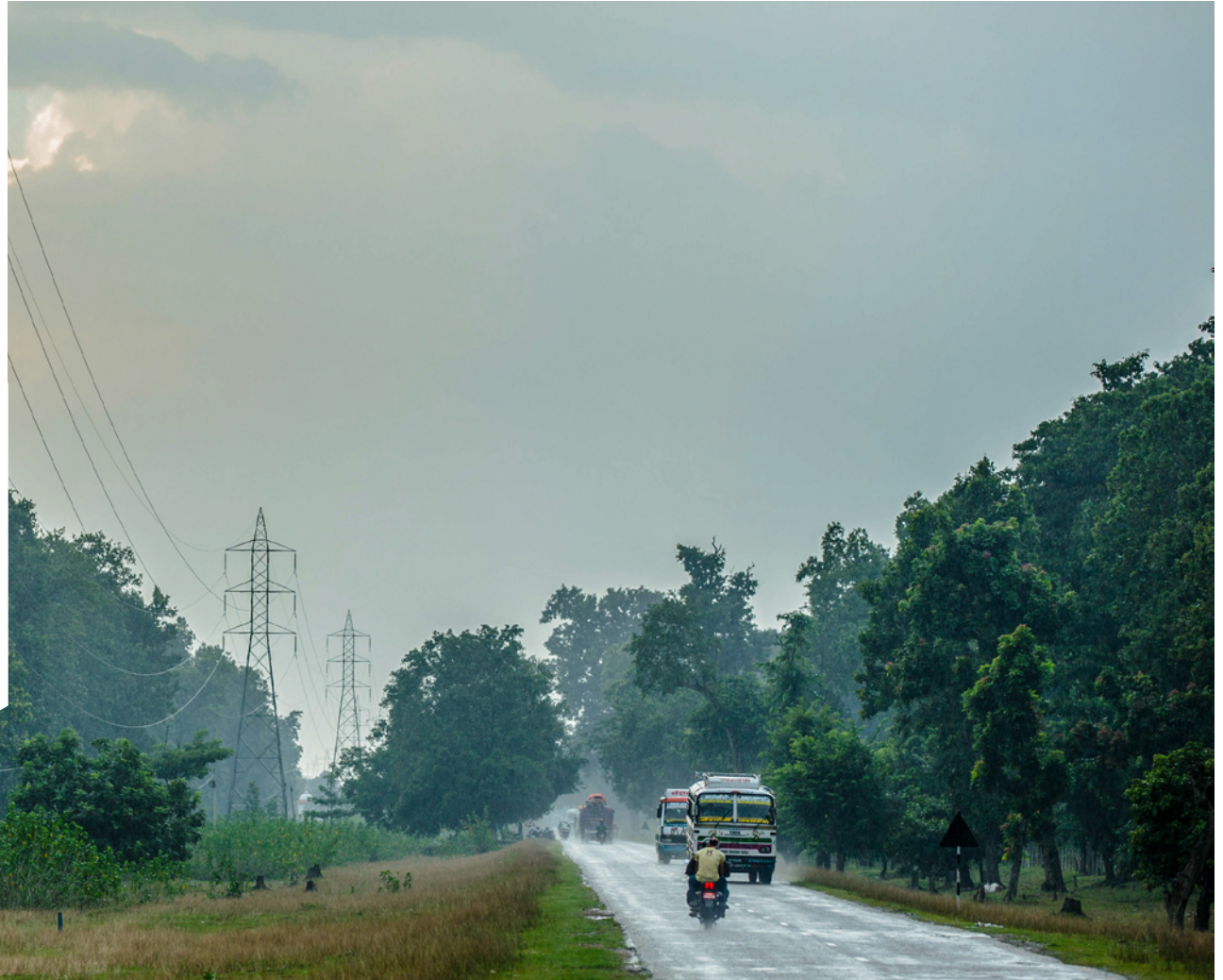
Transmission lines along the Butwal Kohalpur road. PHOTO: ASIAN DEVELOPMENT BANK, 2014
