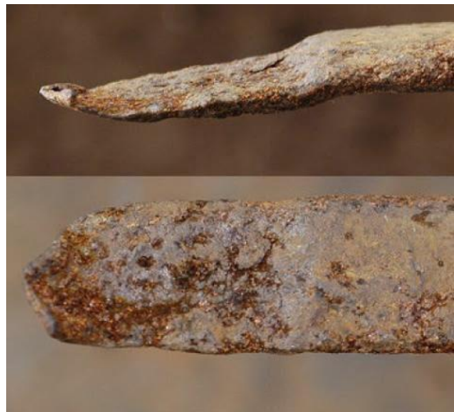
Figure 4-4 Corroded armour wire after breach of external sheath, ref [12]
