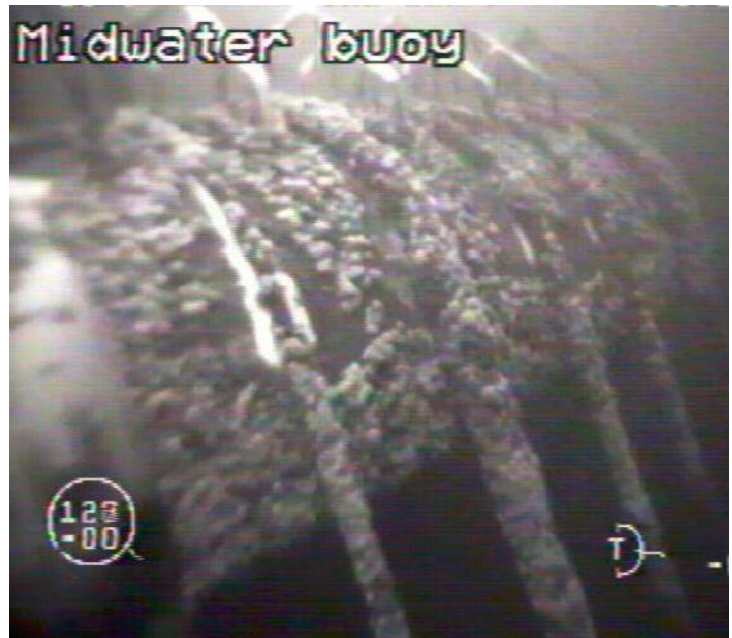
Figure 4-11 Mid-water arch with marine growth (pipe dynamics seen as white areas) (Talisman)
