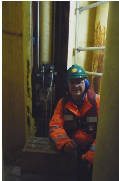
Figure 5-4 MAPS riser inspection inside guide tube, ref [31]
