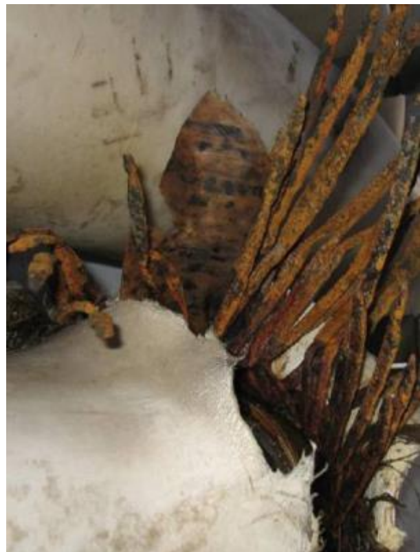
Figure 3-7 Severe corrosion lead to flexible pipe failure in Norway, however not reported as this is not a riser suspended overboard
