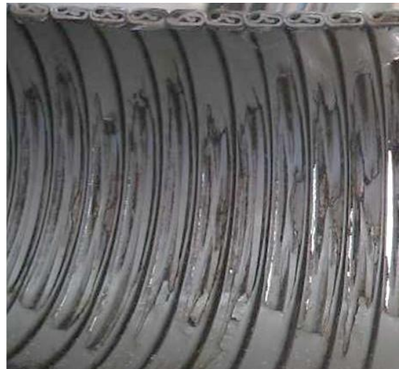
Figure 5-9 Carcass erosion, ref[12]
