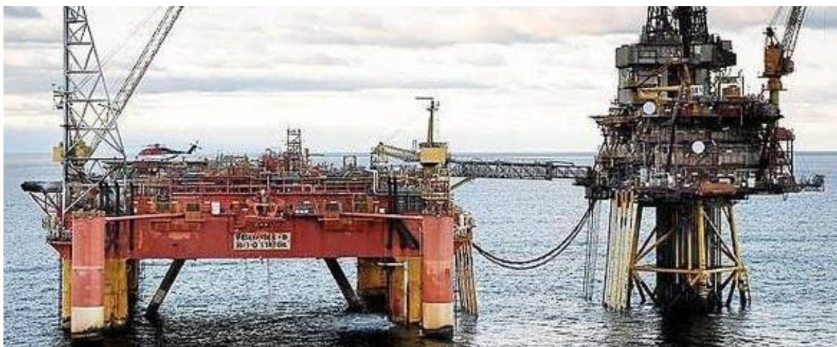
Figure 2-6 Veslefrikk A/B connected by flexible jumpers, bridge and utility lines in air suspension (Statoil)
