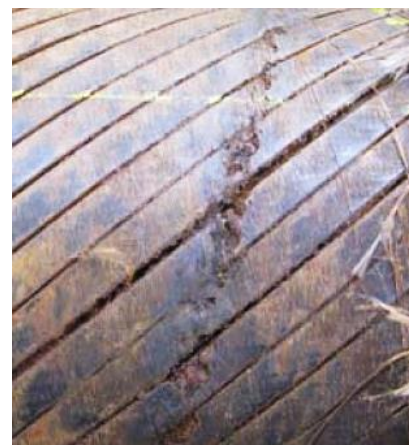
Figure 4-7 Armour wire corrosion (Statoil)
