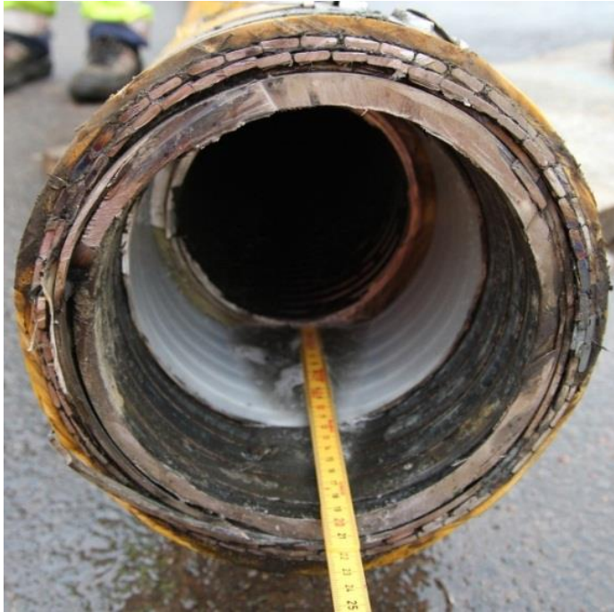
Figure 3-15 Investigation of PVDF shrinkage in a decommissioned flexible riser (4Subsea)
