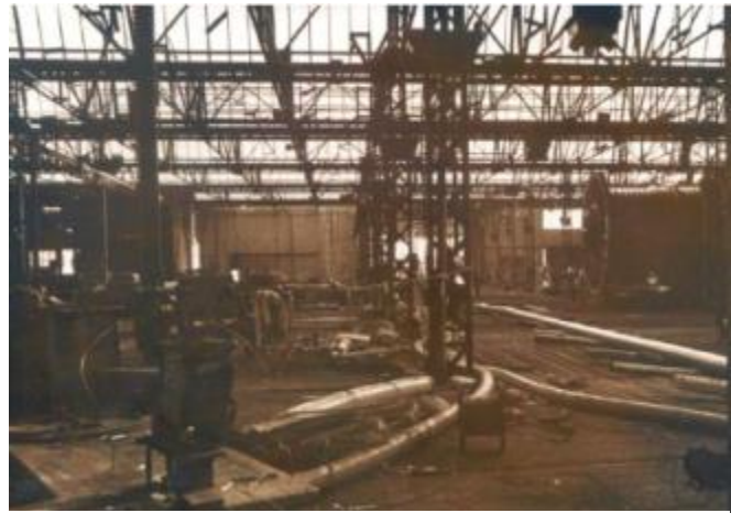
Figure 2-1 An early day in the Bordeaux plant (Technip)
